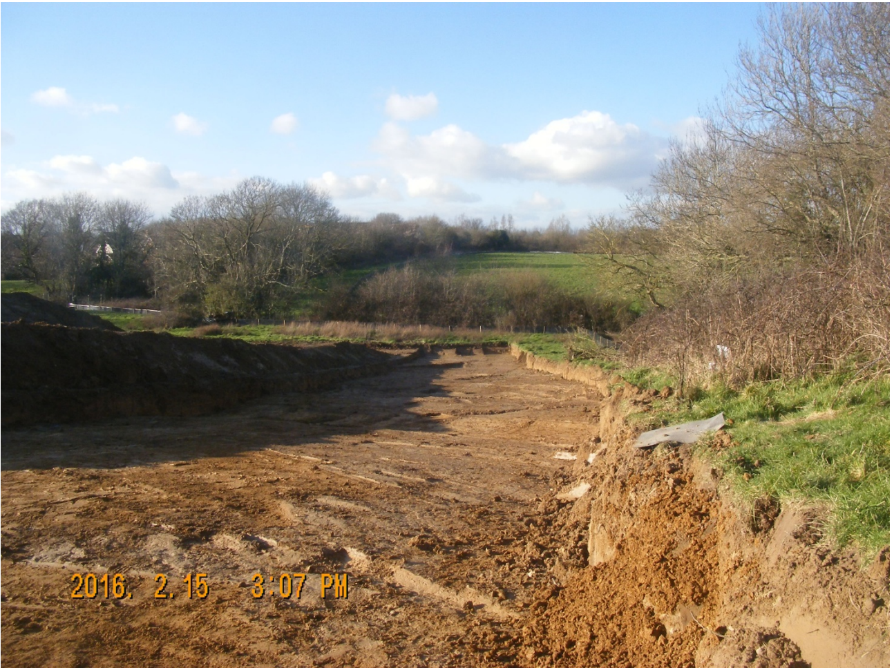
Plate 1: Looking northwest at the area 2 after stripping
